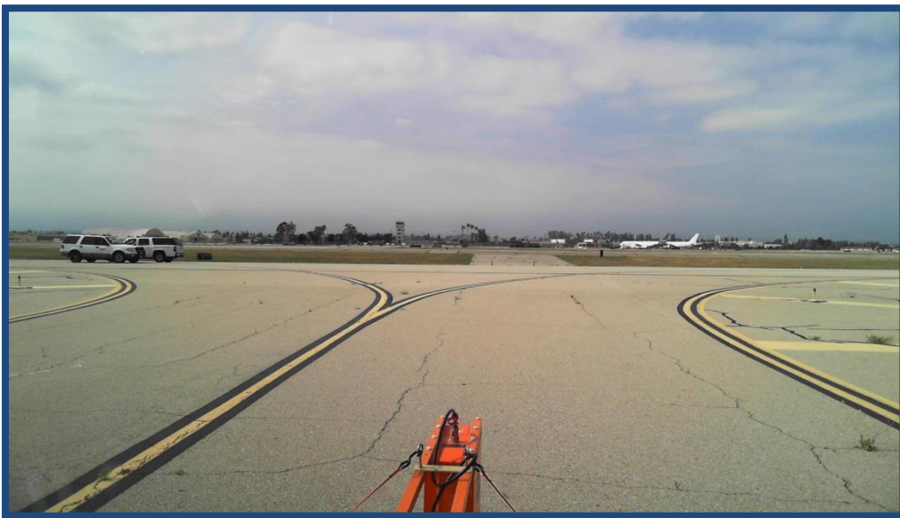
Figure F.21. Taxiway S3 Representative Pavement Condition (Sta. 1+25)
