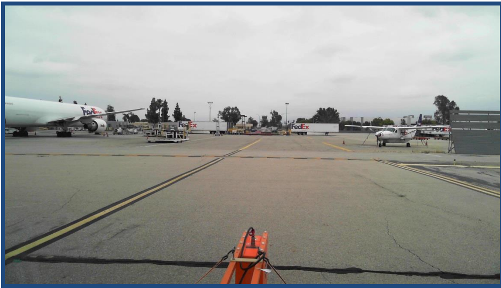
Figure F.19. Taxiway S1 Representative Pavement Condition (Sta. 0+00)
