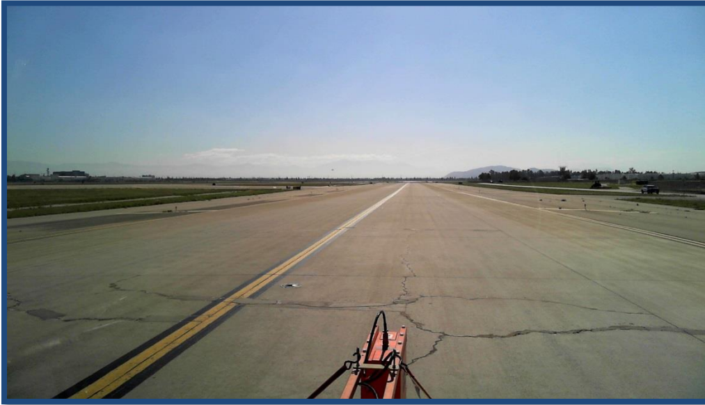
Figure F.6. Taxiway S Representative Pavement Condition (Sta. 46+75)
