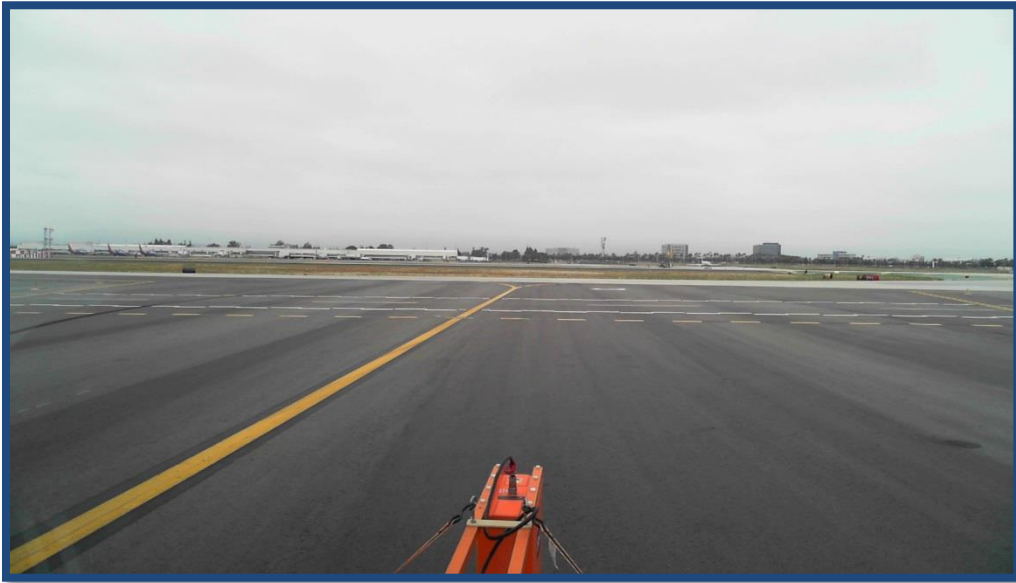
Figure F.22. Taxiway S5 Representative Pavement Condition (Sta. 5+00)
