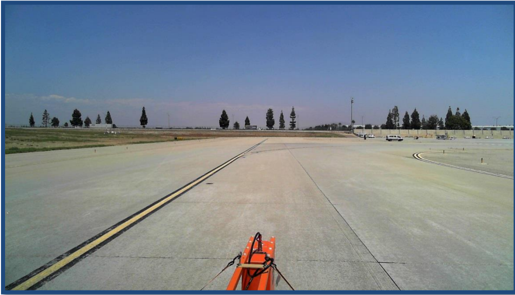
Figure F.30. Taxiway Y Representative Pavement Condition (Sta. 6+87)
