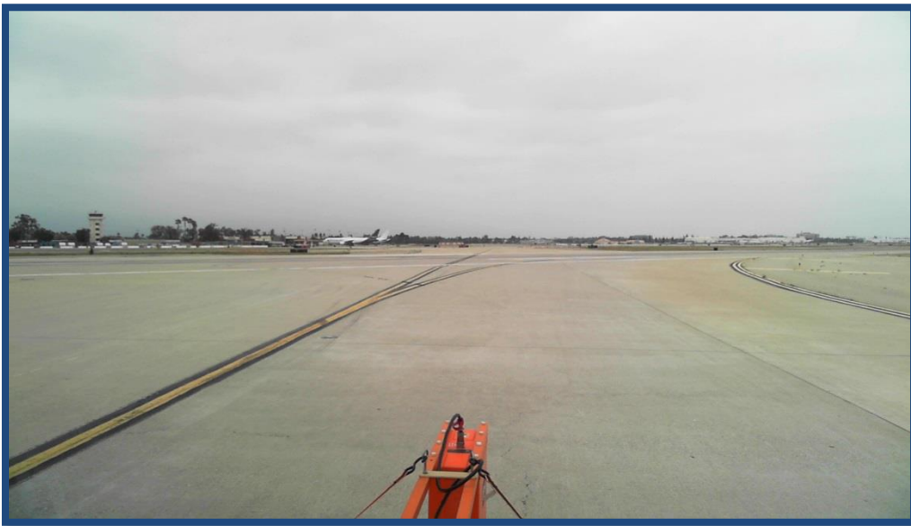
Figure F.11. Taxiway F Representative Pavement Condition (Sta. 2+00)
