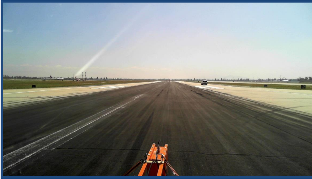
Figure F.2. Runway 8R-26L Representative Pavement Condition (Sta. 23+00)
