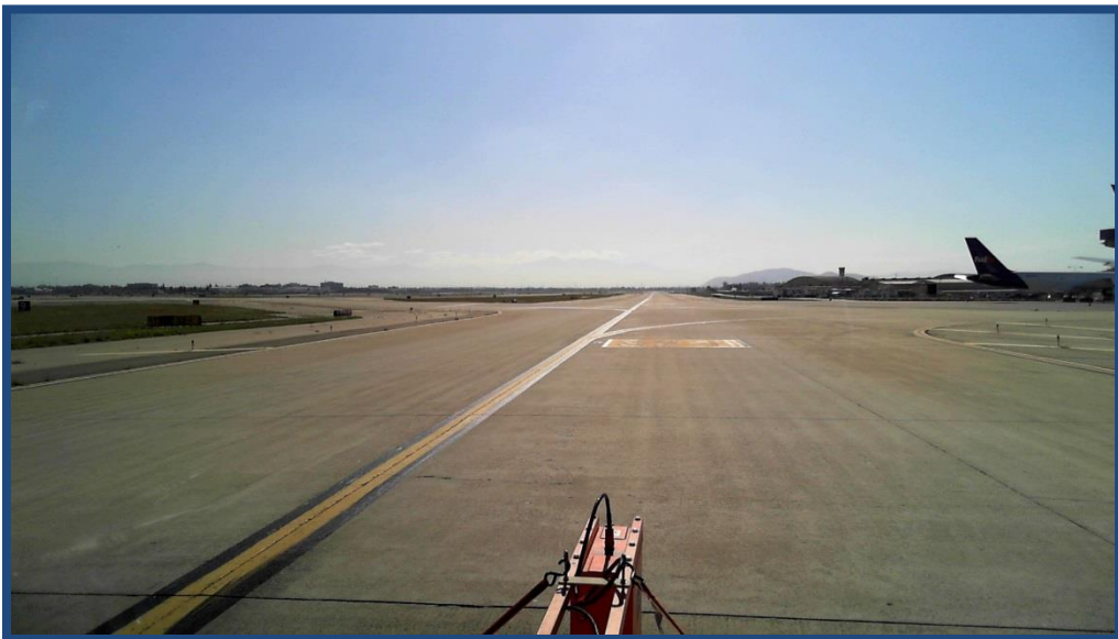
Figure F.5. Taxiway S Representative Pavement Condition (Sta. 6+00)
