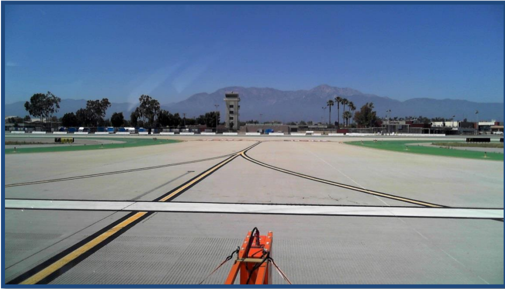
Figure F.12. Taxiway F Representative Pavement Condition (Sta. 3+75)
