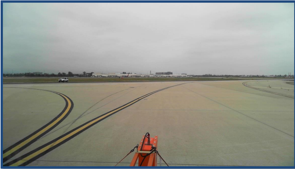
Figure F.24. Taxiway T Representative Pavement Condition (Sta. 1+50)
