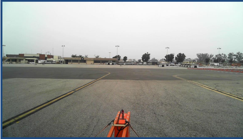
Figure F.42. Taxiway H Representative Pavement Condition (Sta. 0+00)
