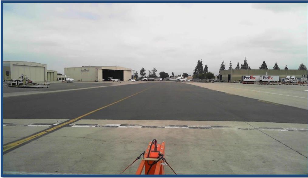
Figure F.20. Taxiway S2 Representative Pavement Condition (Sta. 1+05)
