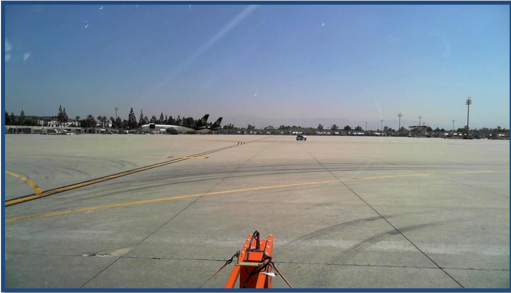
Figure F.32. Taxiway Y2 Representative Pavement Condition (Sta. 1+64)
