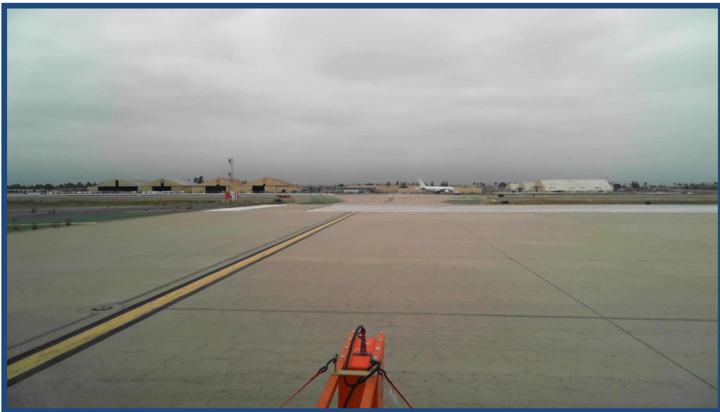
Figure F.9. Taxiway D Representative Pavement Condition (Sta. 2+00)
