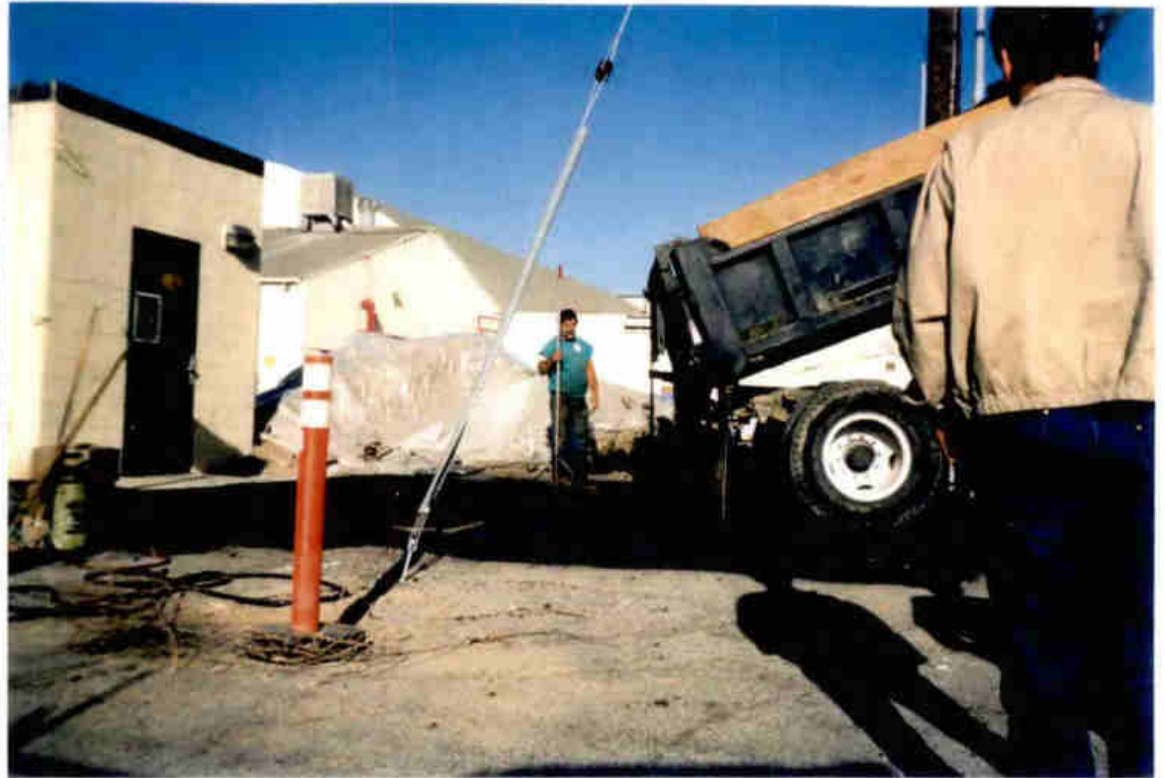
Photo 14. Repaving with asphaltic concrete at Tank 11.
