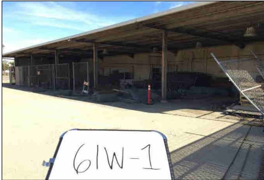
Maintenance shed/scrap yard at the northwest corner of hangar 4.
