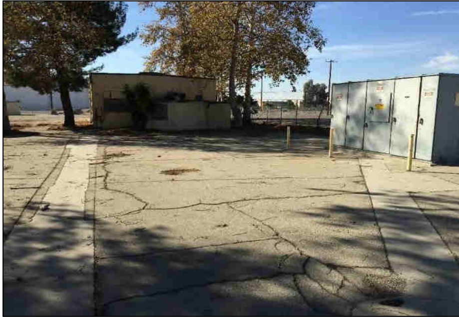
Trenches located inside the maintenance yard.
