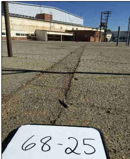
Water line leading to the boiler room.
