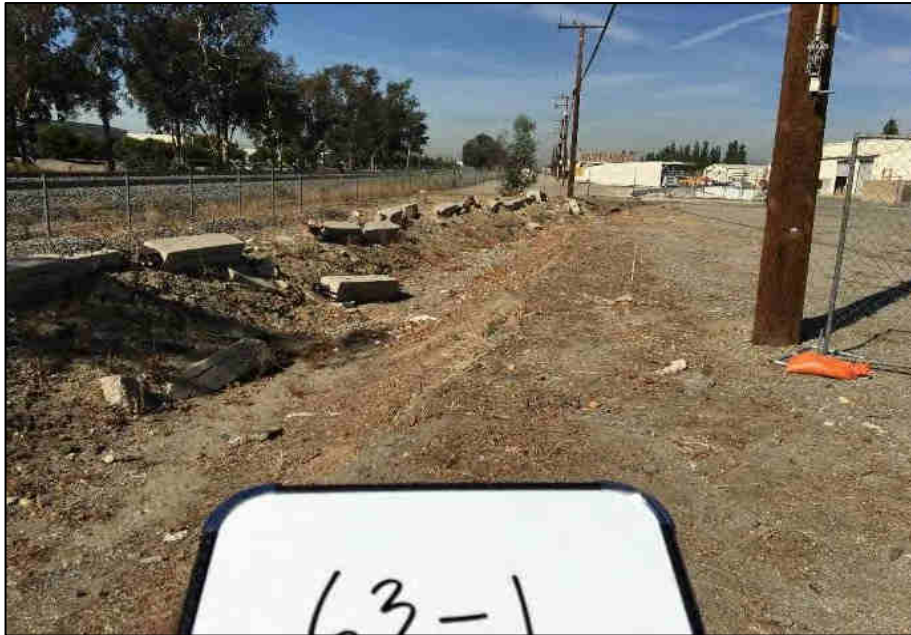
Drainage channel along the southern edge of the Site boundary.
