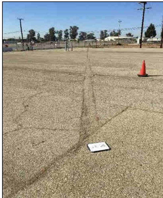
Trench leading to the asphalt patch.
