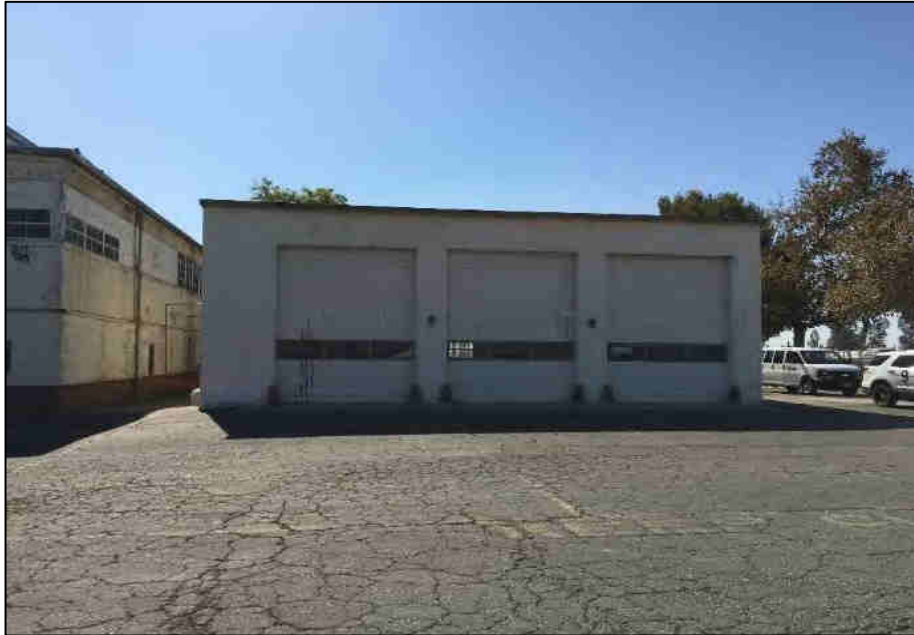
Facing south towards the front of the former Fire House/Auto Shop.
