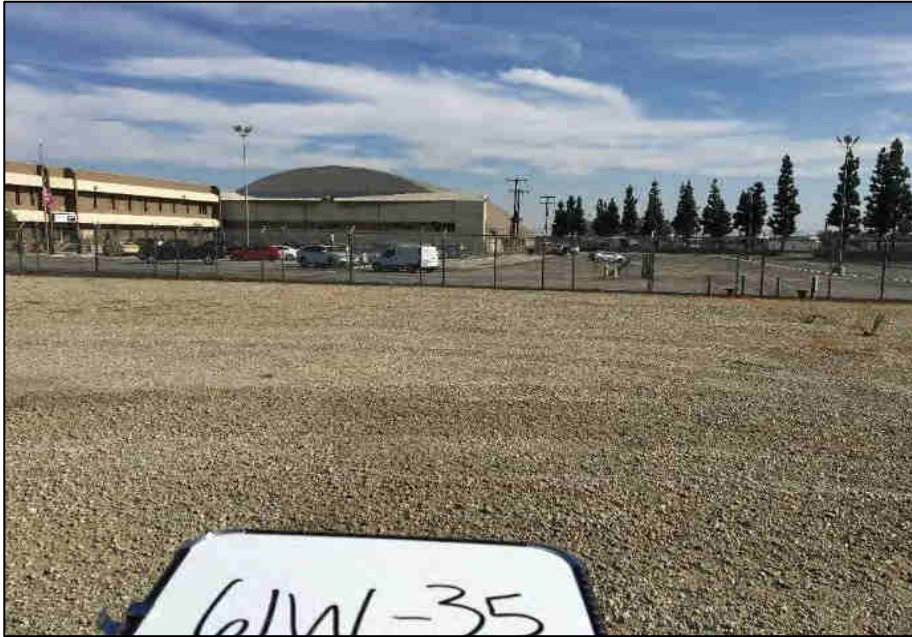
Looking east towards the administration building and hangar 3 from the ASIG dirt lease area.
