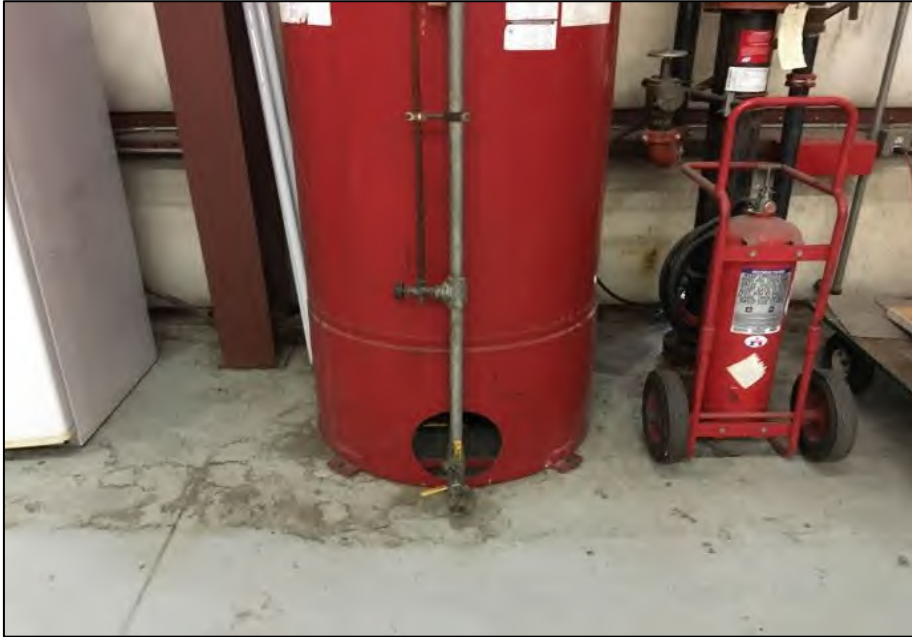
Closer look at staining around the AFFF suppression system.
