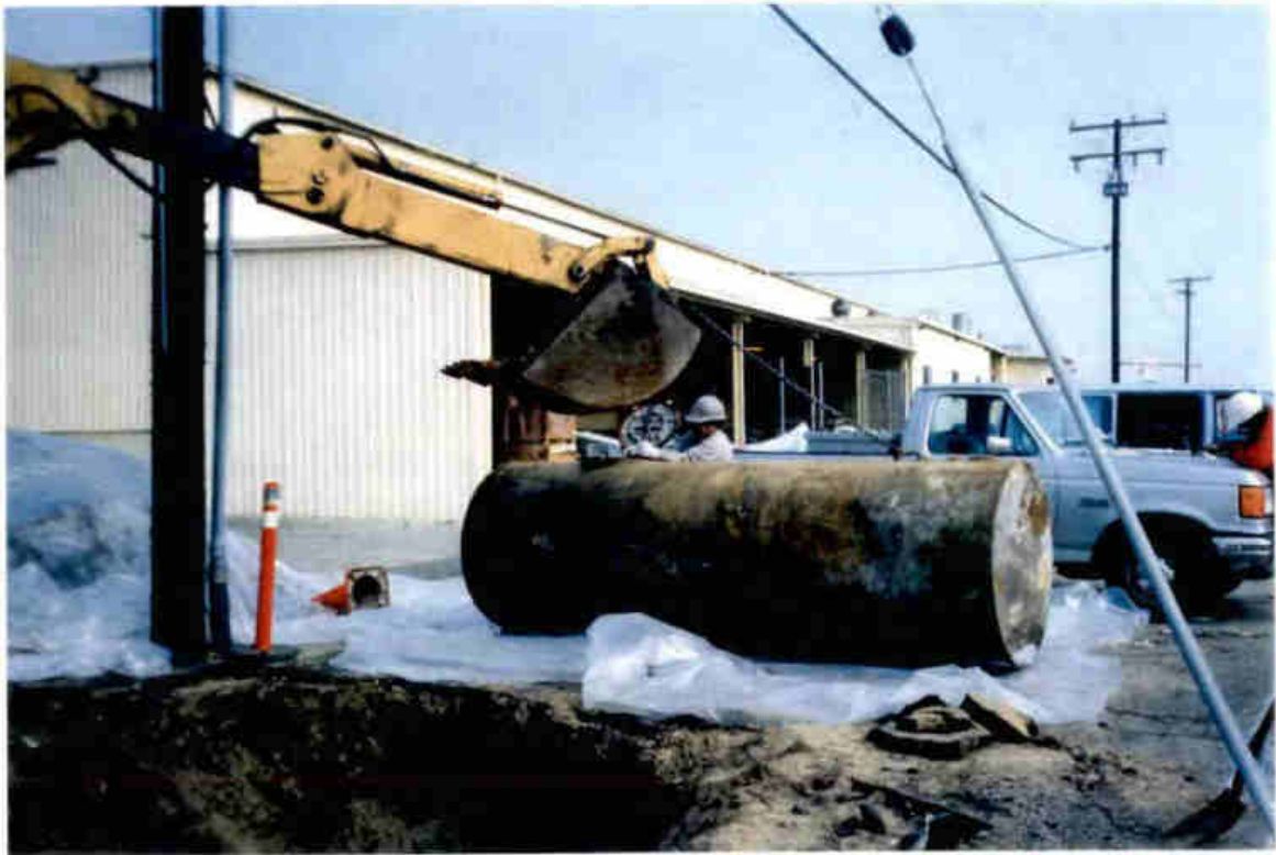
Photo 11. Removing Tank 11 with backhoe.
