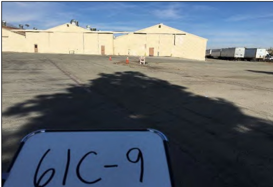
Looking north towards hangar 4 from the parking area.
