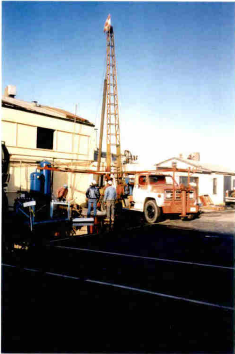
Photo 3. Drilling Beam A for Tank 9, north side of Flow Room Building.
