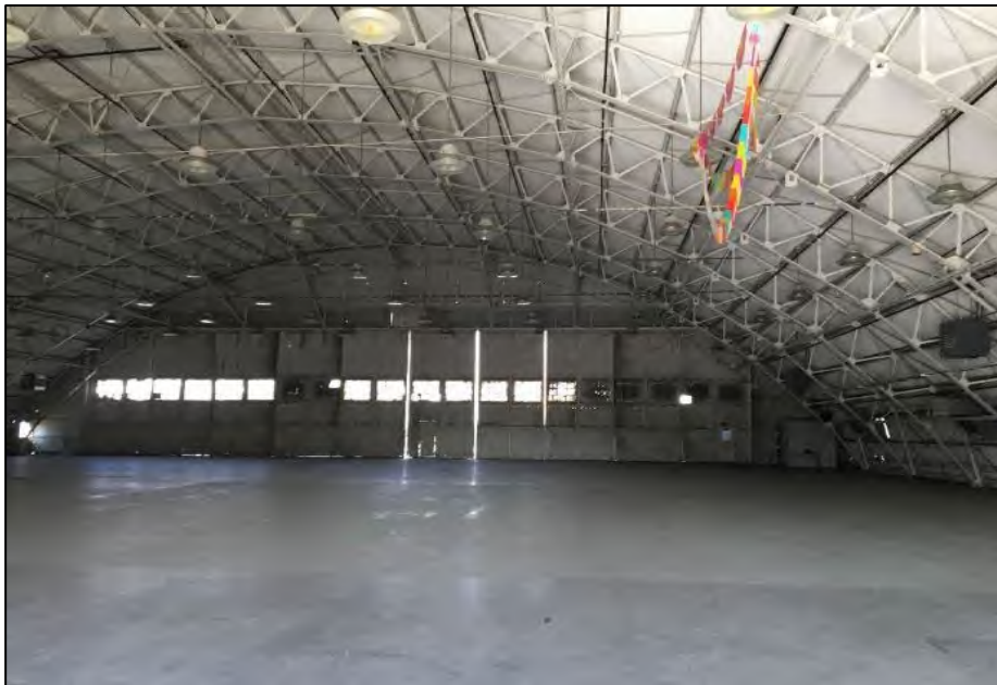
Looking inside of hangar 3.
