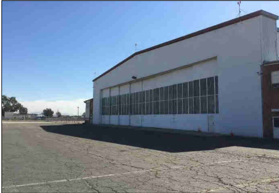
Facing south towards the front of the former CANG hangar.
