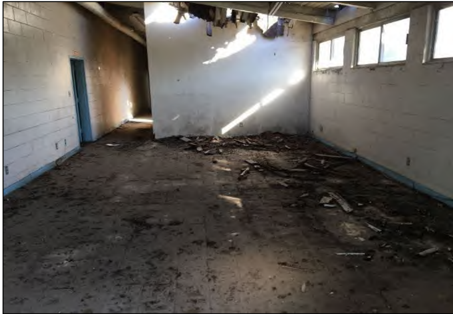
Inside of the first building.
