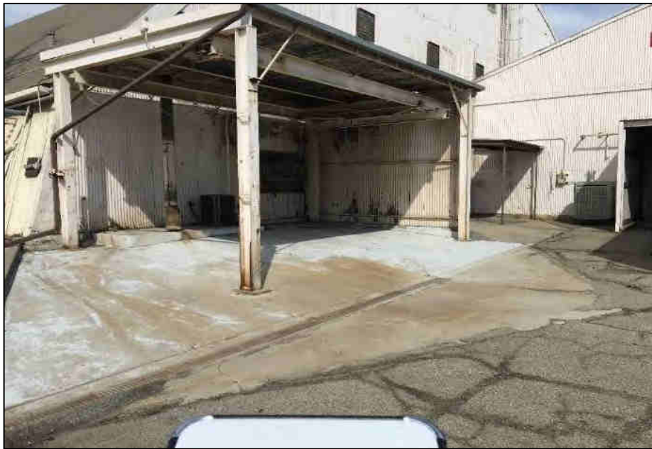
Trench drain located southwest of hangar 2 below a sloped concrete patch and awning.
