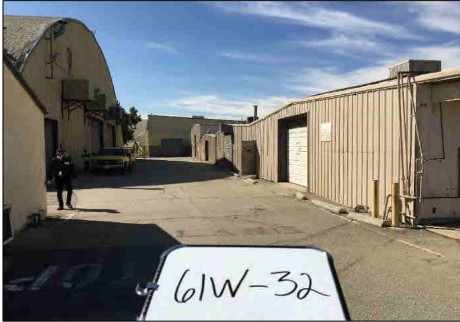
Facing south towards the building west of hangar 1.
