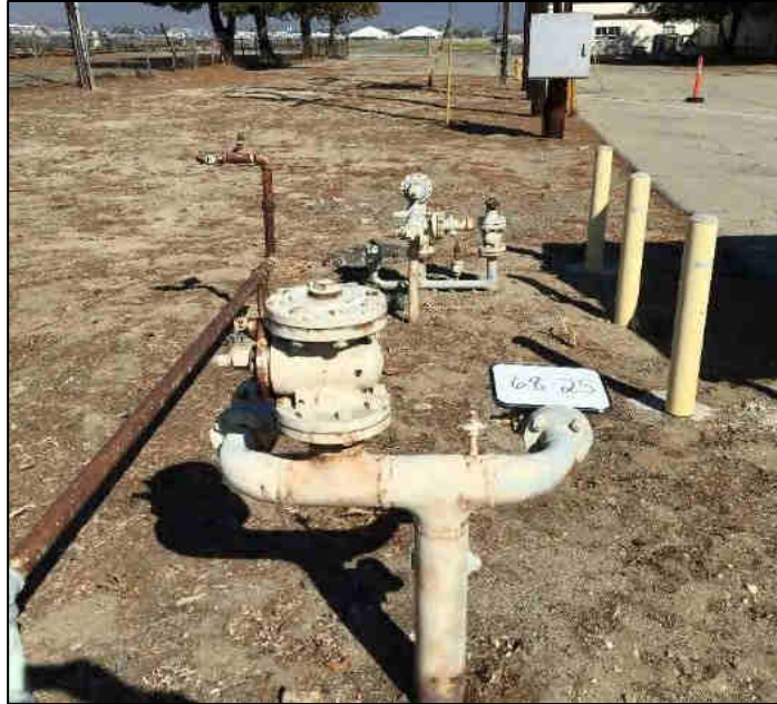
Water source that leads to boiler room located south of 68-21.
