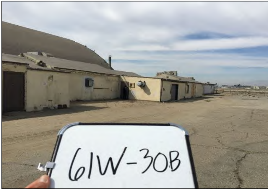
Facing south towards the ancillary structure next to the garages.
