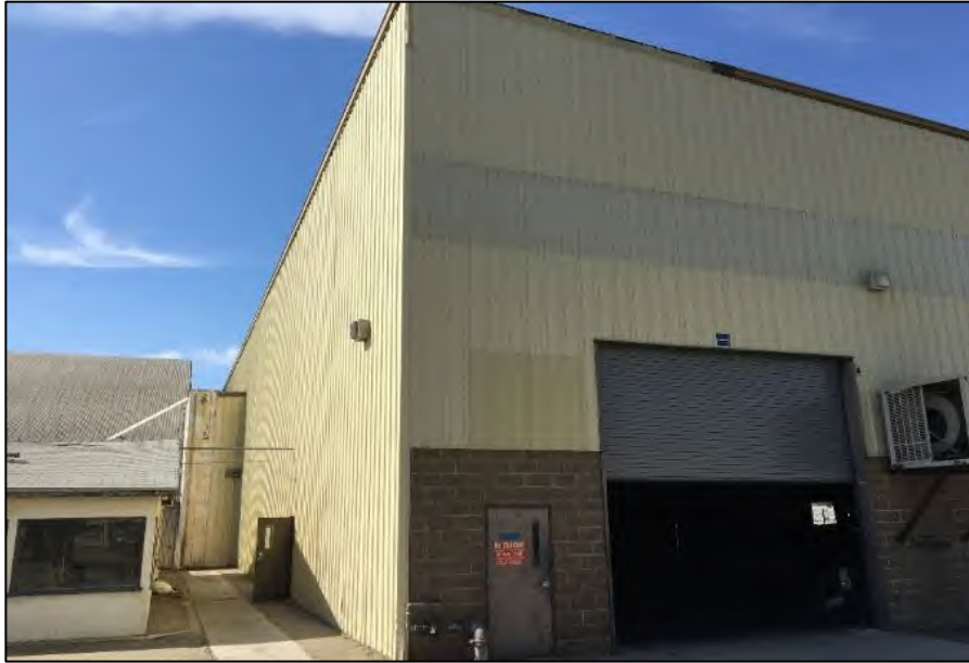
Facing south towards the administration building and adjacent hangar 2.
