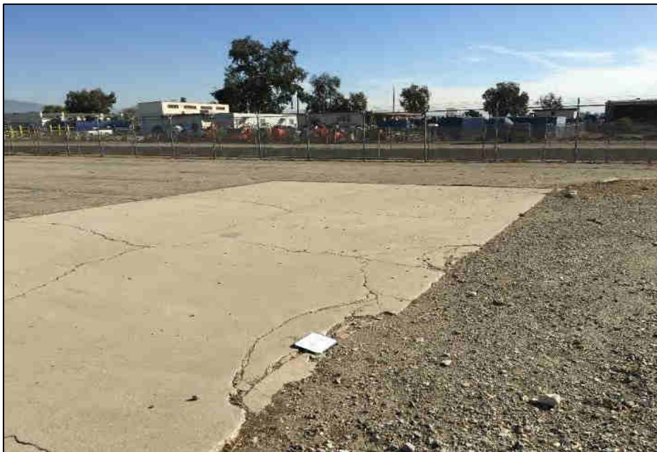
Concrete pad north of concrete pad discussed above.
