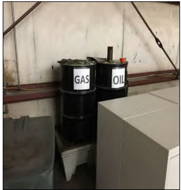
Oil and gas drums inside the Guardian Center southern hangar with no bungs, absorbent pads and used oil filters.
