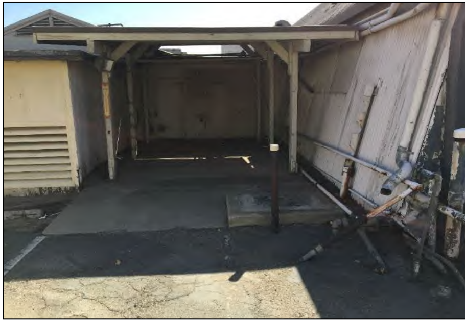
Ancillary awning north of hangar 1.
