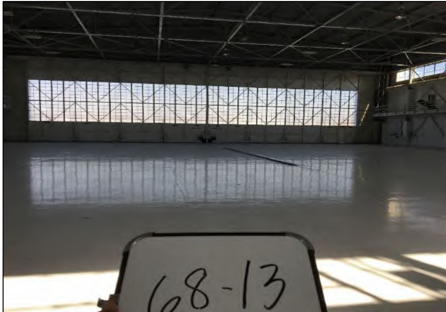
Inside of the CANG hangar.
