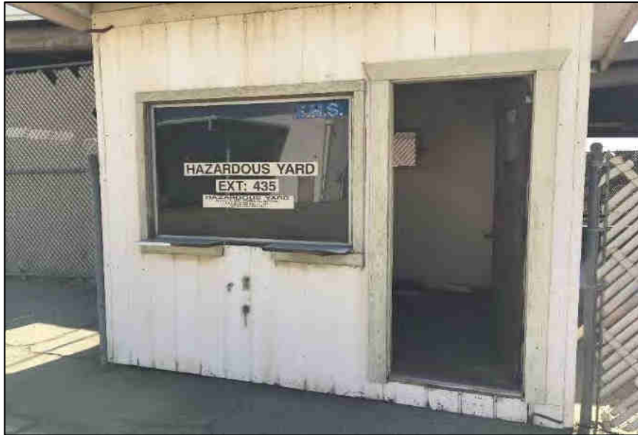
Hazardous waste storage structure south of hangars 2 and 3.
