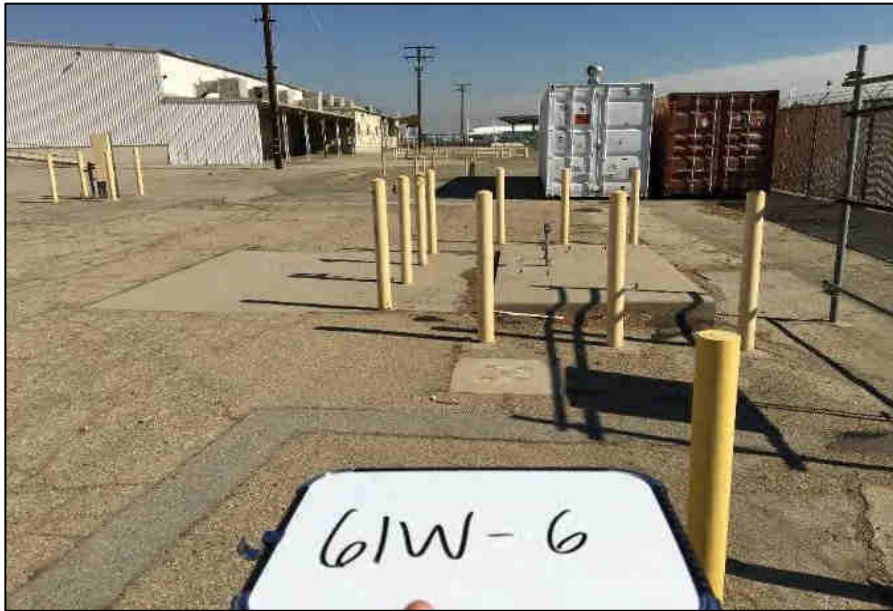
Facing north towards a concrete pad where propane ASTs used to be stored.
