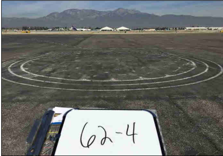
Helicopter pad to the east of the Guardian East hangar.
