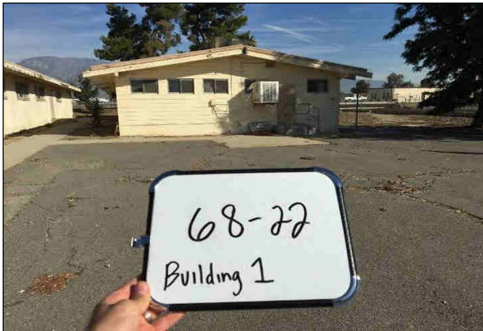
Facing north towards the most eastern building in the maintenance yard.
