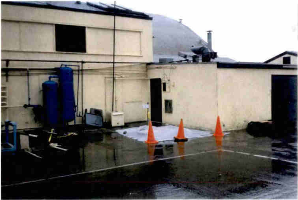
Photo 1. 7,000 - Gallon Calibration Fluid (Tank 9) before excavation.
