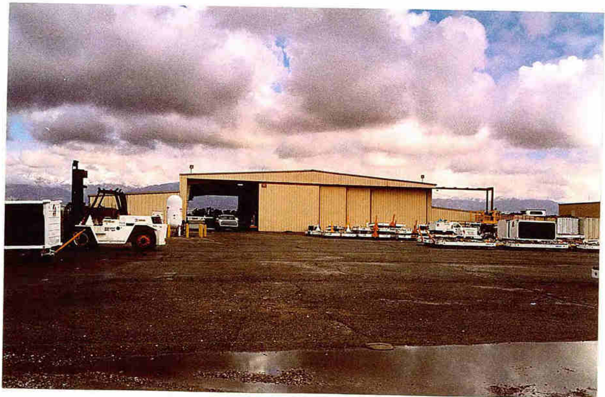
2. View of Building 2, looking toward the north.
