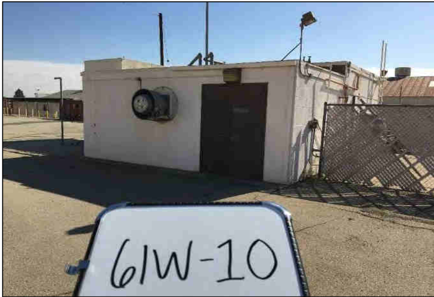
Electrical building east of the elevated storage shed.
