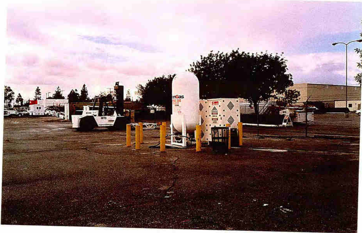
5. Propane AST located to the south of Building 2.
