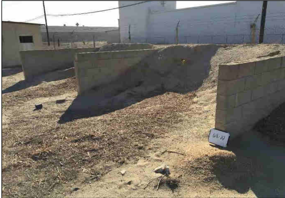
Stockpile bays full of sand inside the maintenance yard.
