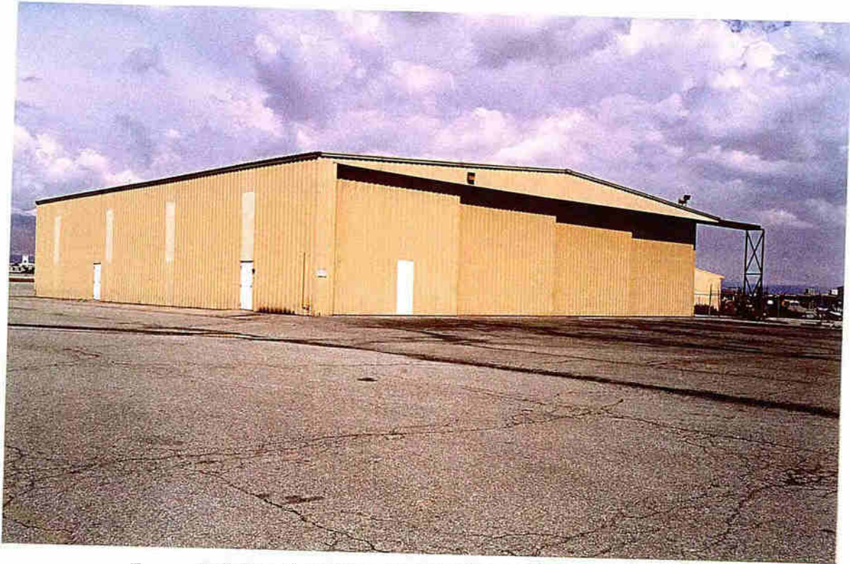
7. Building 3, looking toward the northeast.
