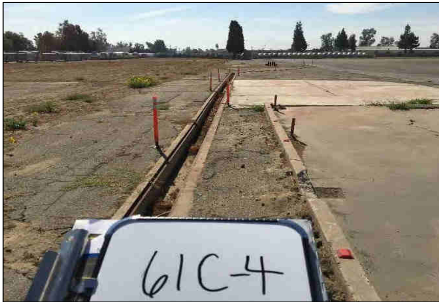
Drainage channel along a former wash rack to the east of the Guardian Jet Center hangars.
