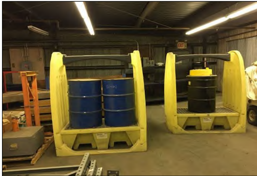
Inside of 61W-32, building #3. Diesel drums and a waste coolant drum in secondary containers.
