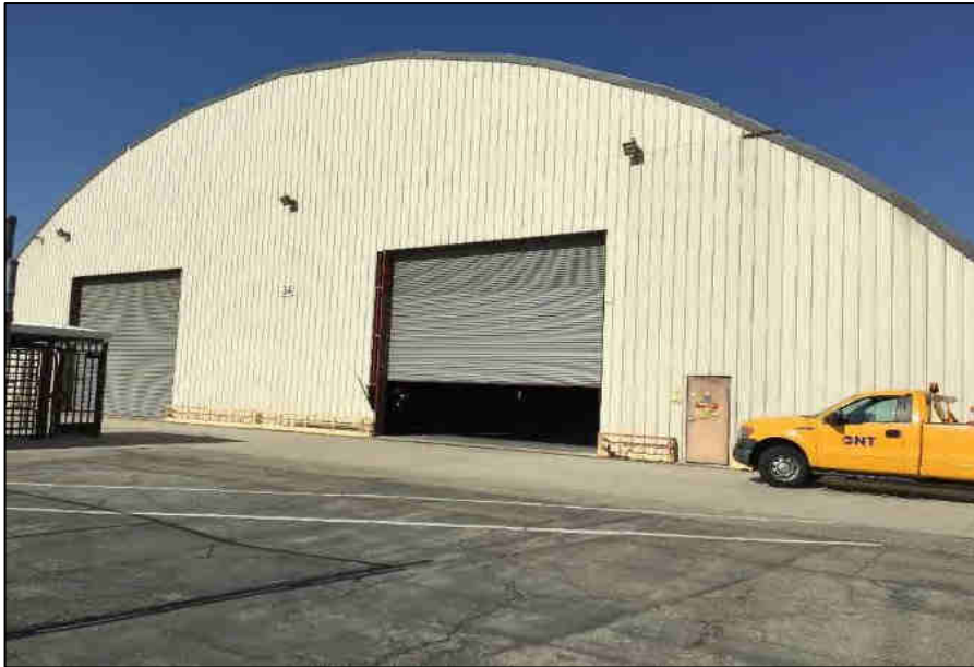
Facing north towards the rollup doors of hangar 3.
