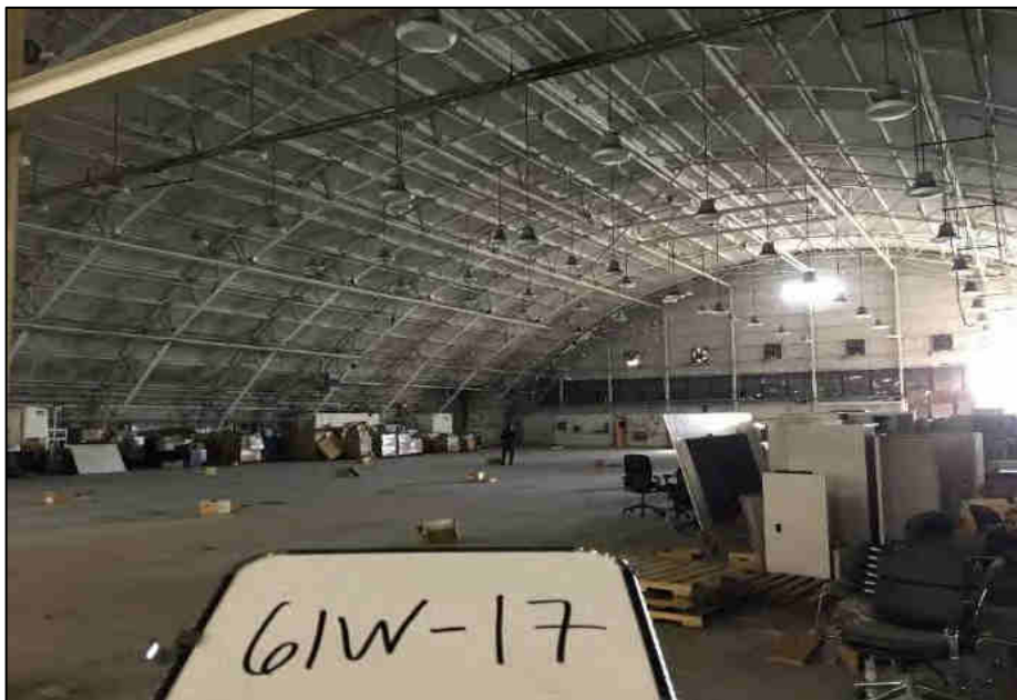
Looking inside of hangar 2.
