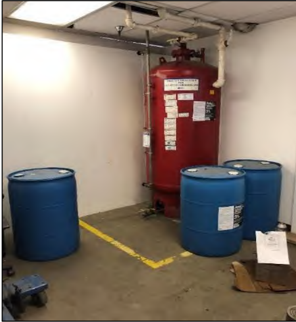
AFFF suppression system found inside Guardian East hangar. Dripping visible on second photo.
