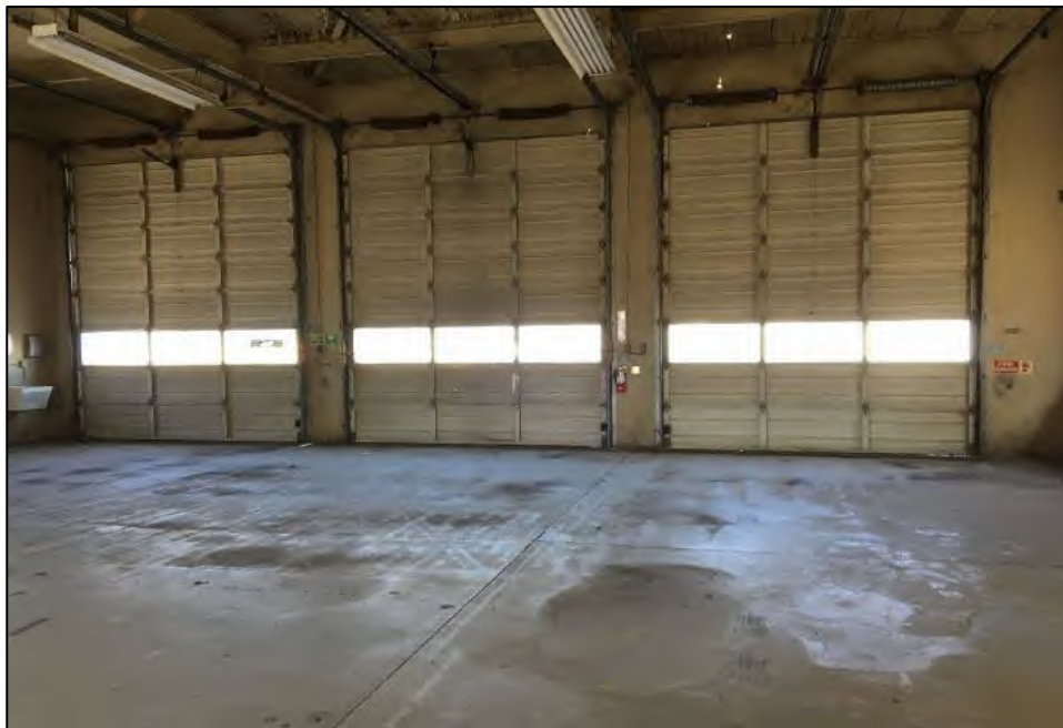
Inside the Fire House/Auto Shop.
