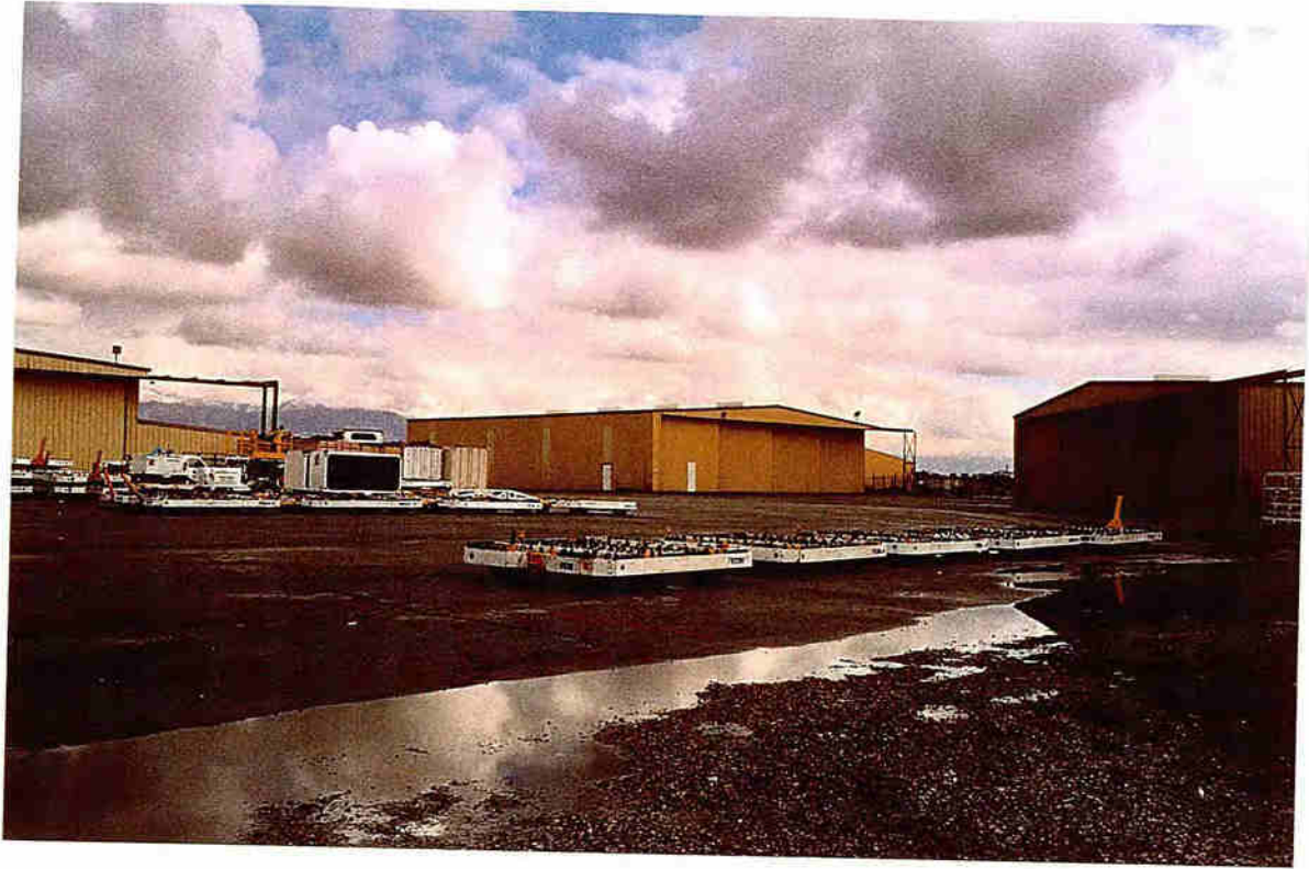
1. View of the subject property, looking toward the northeast.
