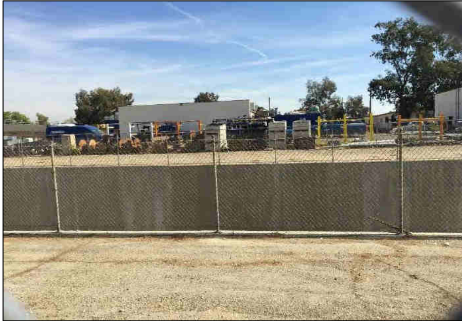
Surrounding property to the east of the Site Boundary-Former wash rack and generator maintenance area.
