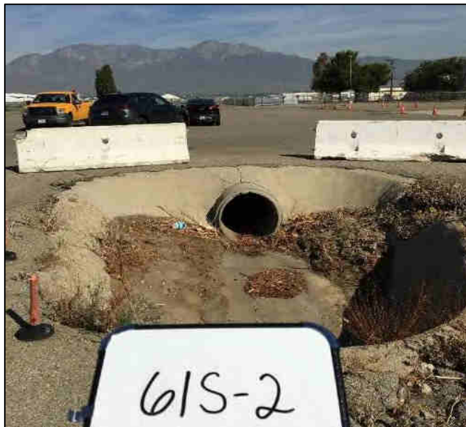
Looking at a storm drain in the southern portion of Parcel 61.
