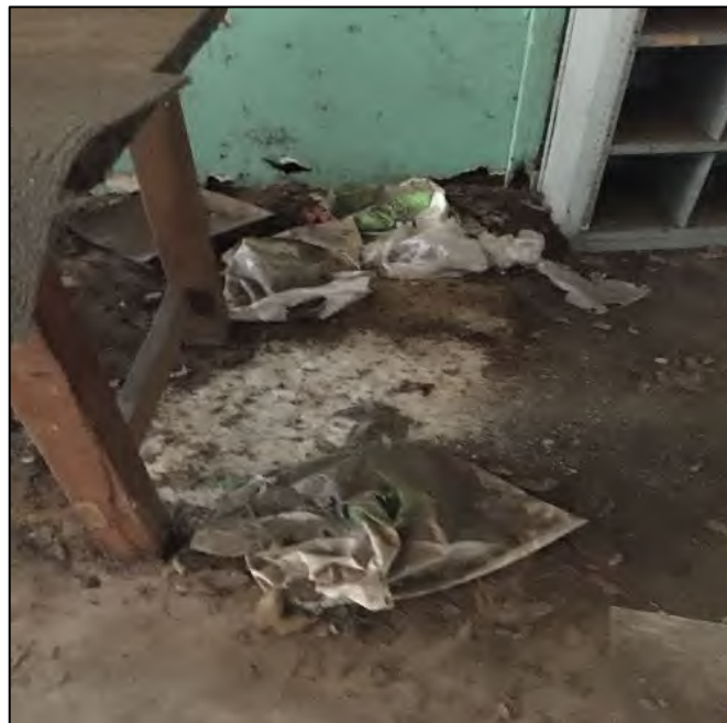
Close up of spilled fertilizer bags inside of 68-22 Building #3.
