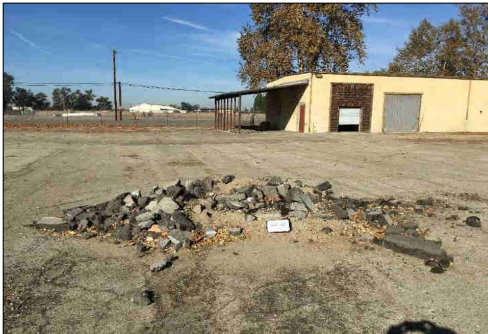
Stockpile of asphalt inside the maintenance yard.
