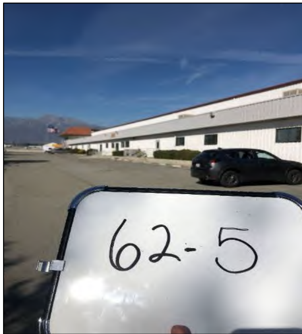
Looking at the western side of the Guardian East building.
