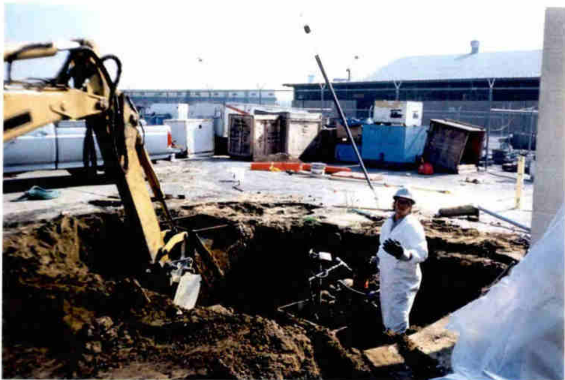
Photo 6. Excavating Tank 11. Pump assembly located in manway to right.
