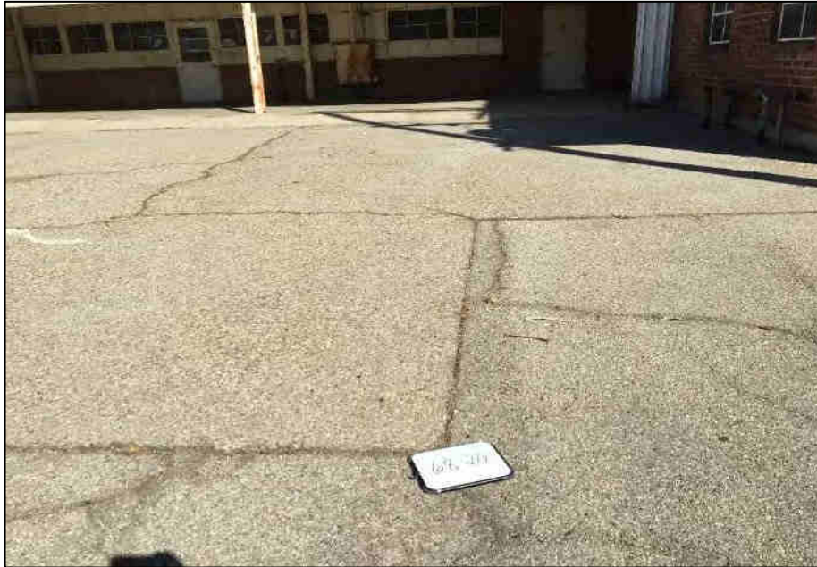
Backfilled asphalt patch to the west of the boiler room.
