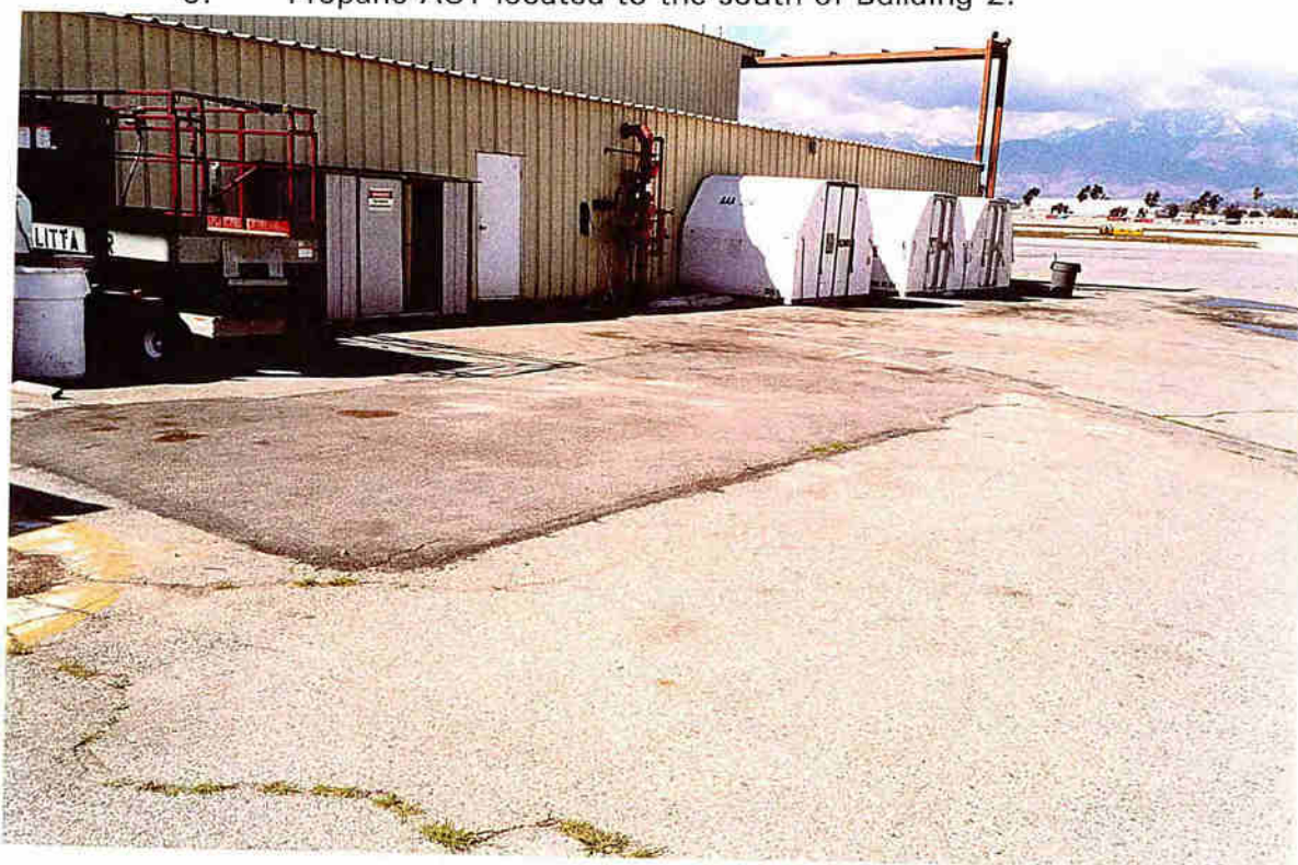
6. Former UST location at the east side of Building 2.
