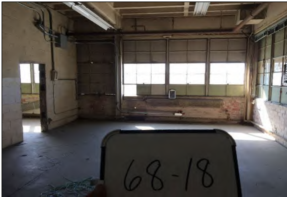
Inside of the building connected to the awning.
