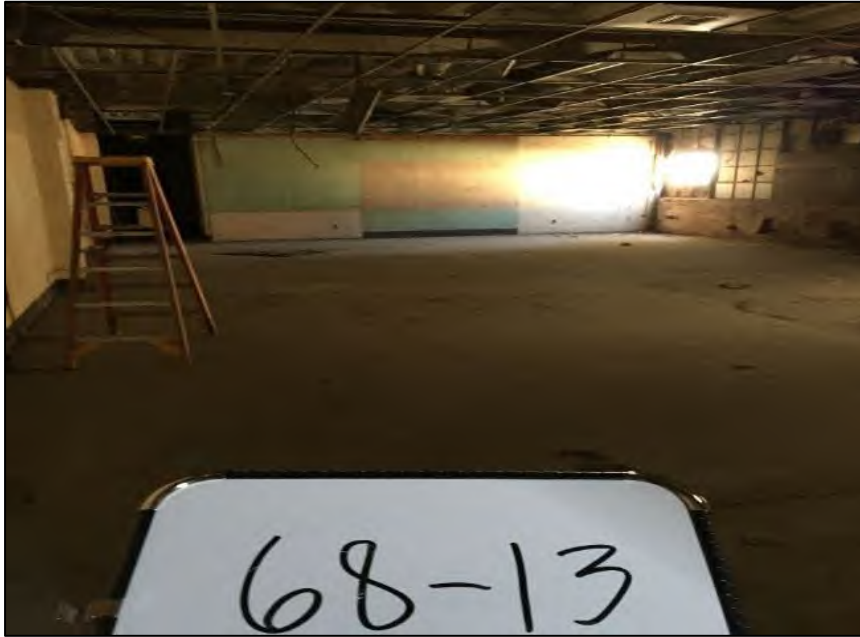
Inside of the operations building.
