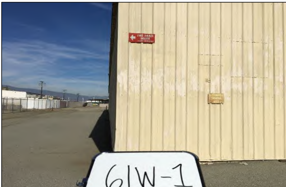
Outside of the structure to the southwest of hangar 4 where a Hazardous Storage sign is located.
