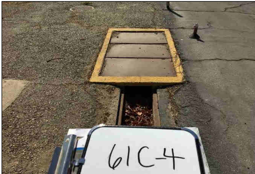
Possible 3 stage clarifier that drainage channel leads to.
