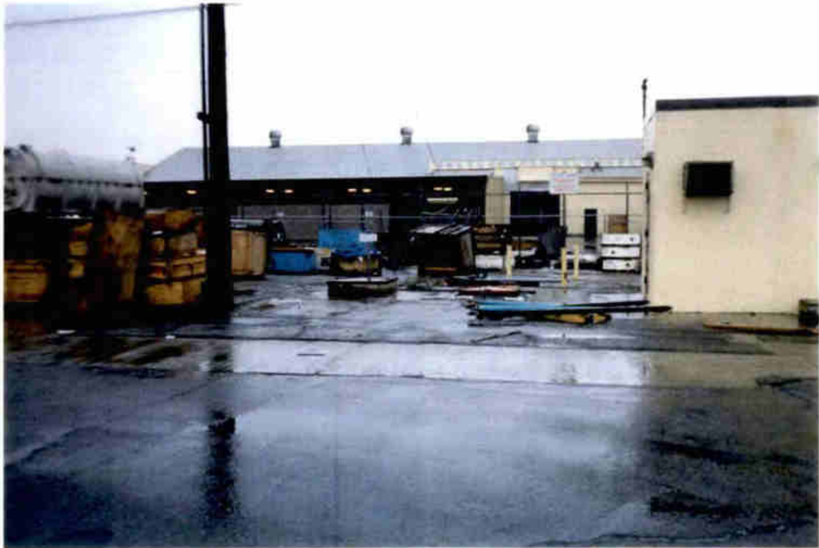
Photo 2. 1,000 - Gallon Jet A Fuel (Tank 11) before excavation.
