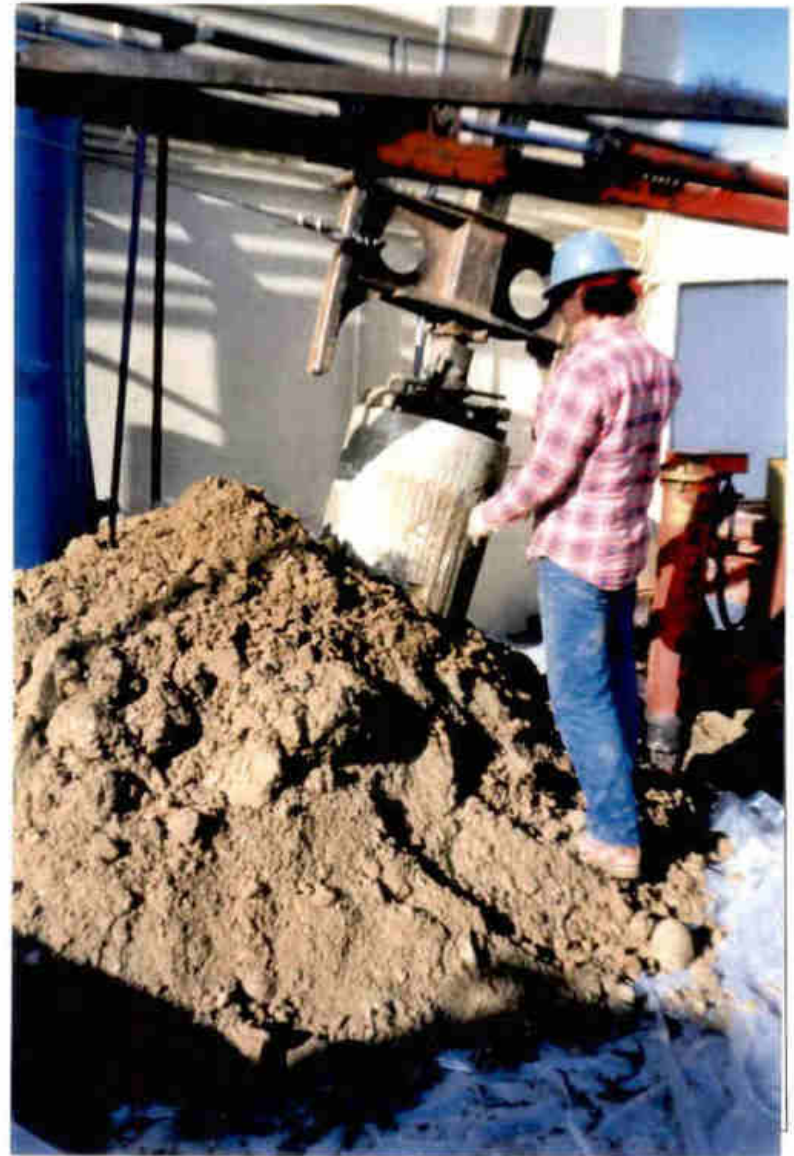
Photo 4. Soil cuttings from drilling Beam A at Tank 9. 20-inch bucket pictured.
