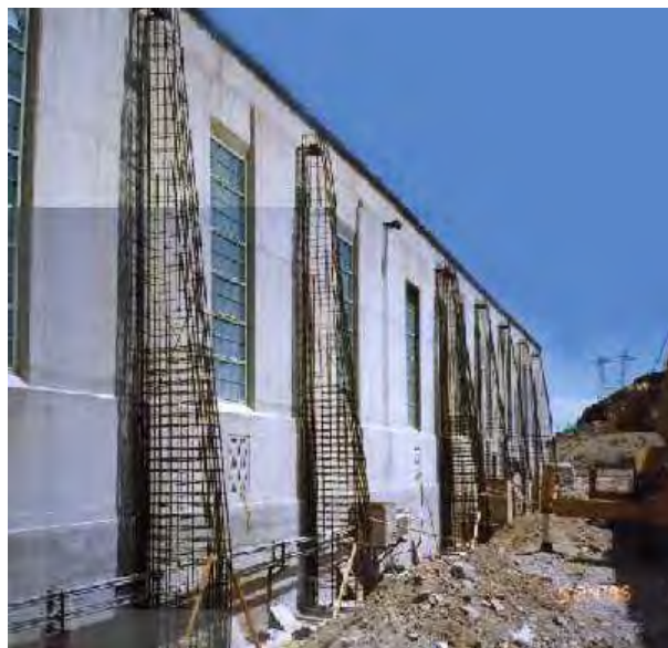
Construction of new buttress walls at Hinds Pumping Plant
