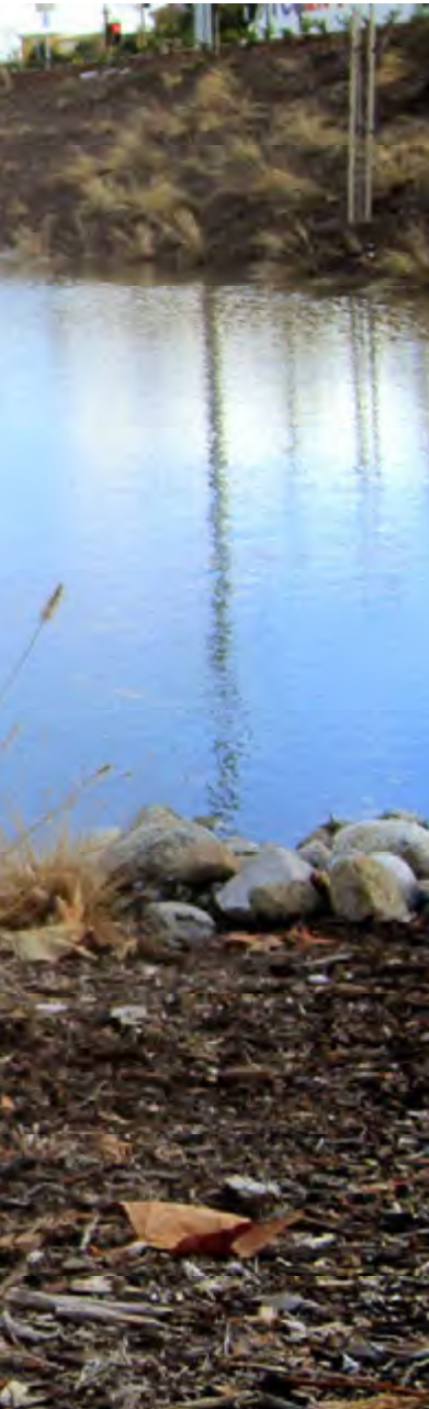
A bio-swale slowly infiltrates stormwater runoff after a winter rain event in the City of Chino.
