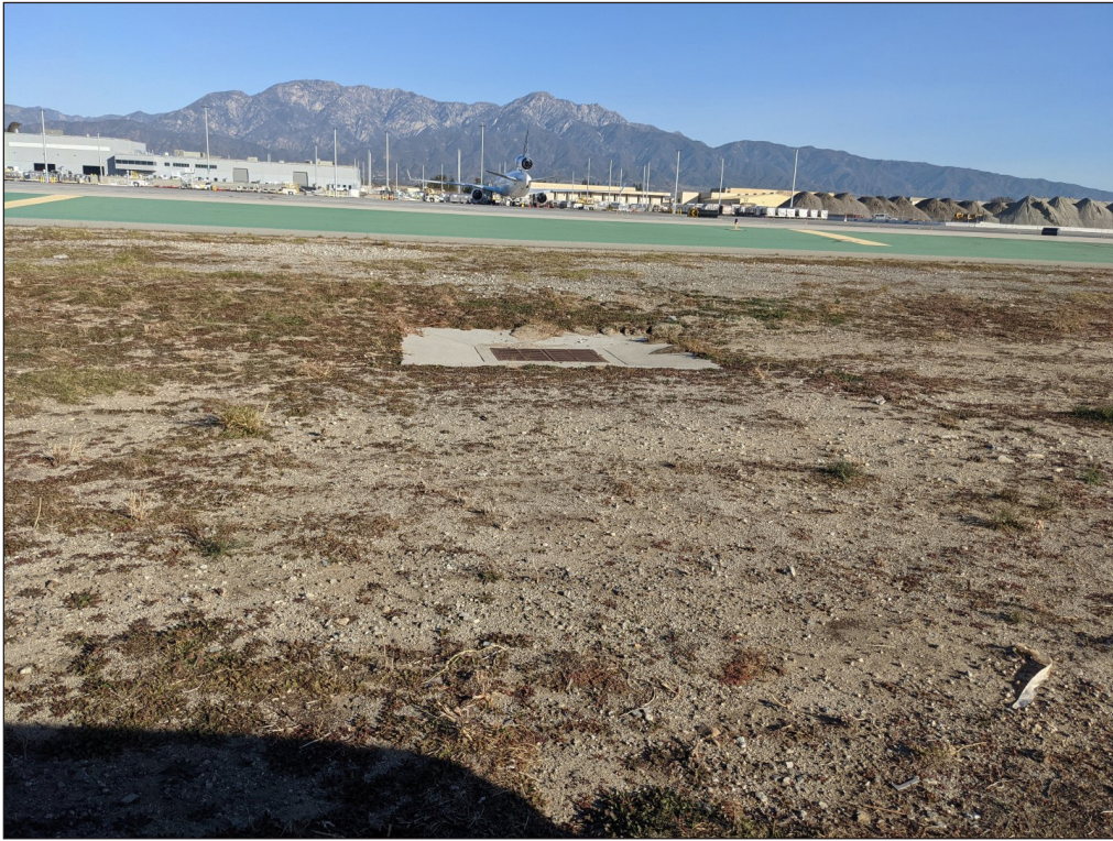
Photo 3: One of several storm drains on the project site leading to a concrete lined channel running under the airport property.
